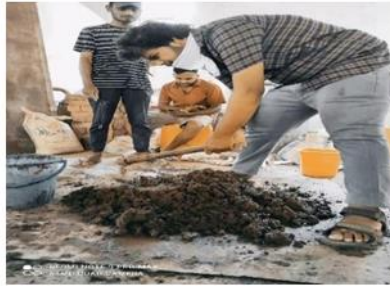
Dry mixing of materials
