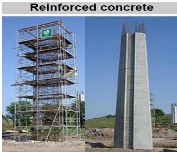
Figure 1: Before and after the concrete was placed in place around the rebar cage of a massive reinforced concrete column
